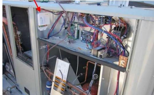
The COOLNOMIX® temperature setpoints are determined at installation and settings do not need to be changed if the setpoints are increased (i.e. during setbacks). If setpoints are decreased, COOLNOMIX® setpoints may be modified to maximize savings opportunities.
